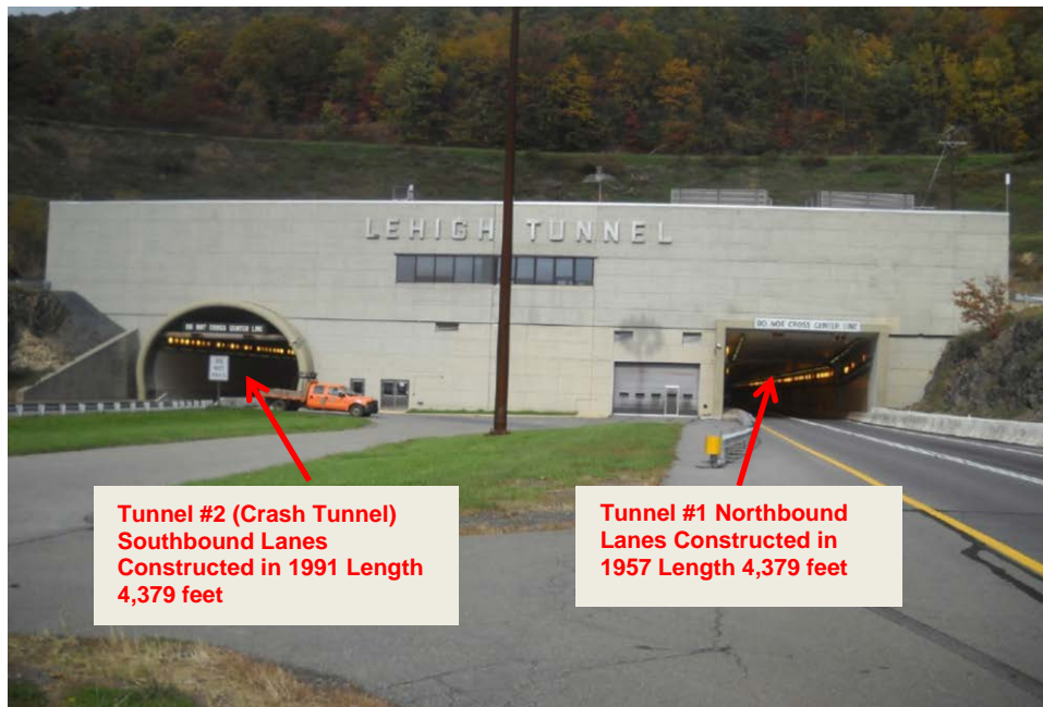
Figure 1. Photograph of the Lehigh Tunnel south portal entrance. The crash occurred in the southbound (left) tunnel.
