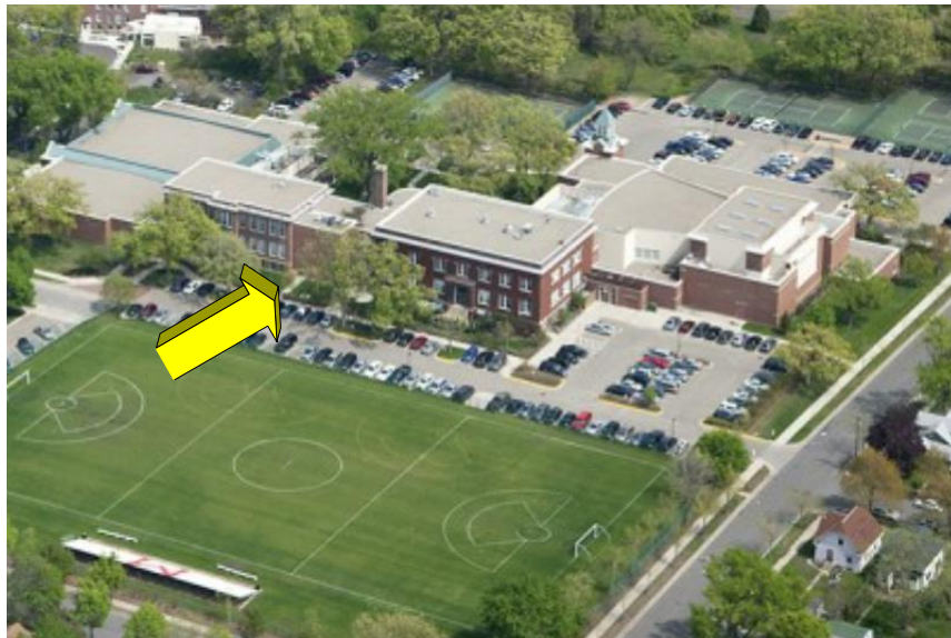
Figure 1. Aerial view of Minnehaha Academy; yellow arrow indicates area of explosion. (Photo courtesy of minnehahaacademy.net)
