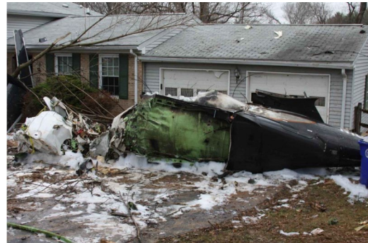
Figure 1. Fuselage showing impact and fire damage to house.
