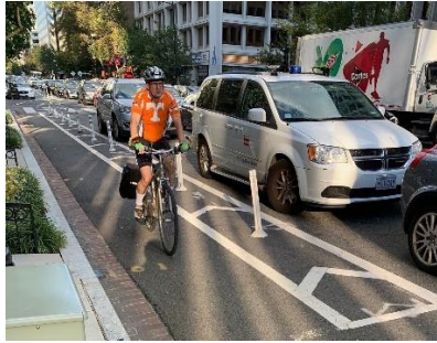
b. One-way separated bike lane with parking as barrier
