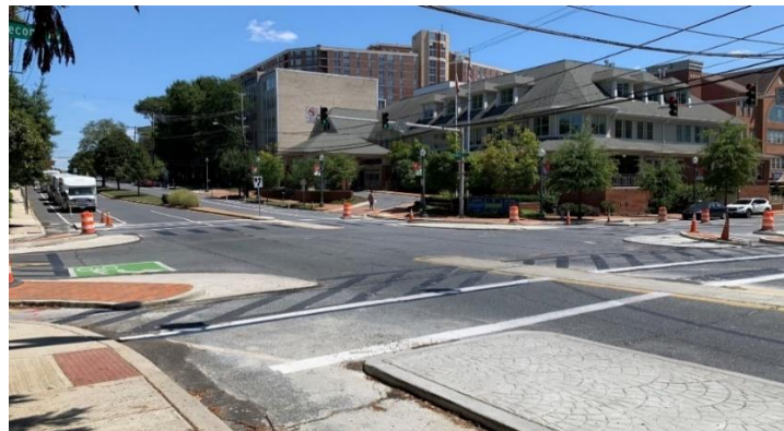
f. Protected intersection with four islands that (1) separate right-turning bicycles from motor vehicles and (2) position left-turning bicycles along the pedestrian crossing facing the traffic signal
