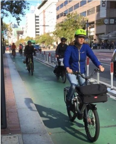
a. Painted one-way separated bike lane with vertical barrier
