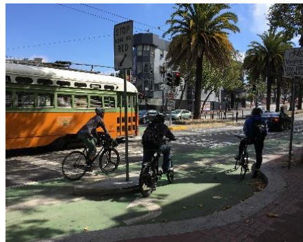
e. Two-stage bicycle turn box with bicycle signal face
