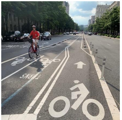
e. Two-way separated bike lane with vertical barrier (center of roadway)
