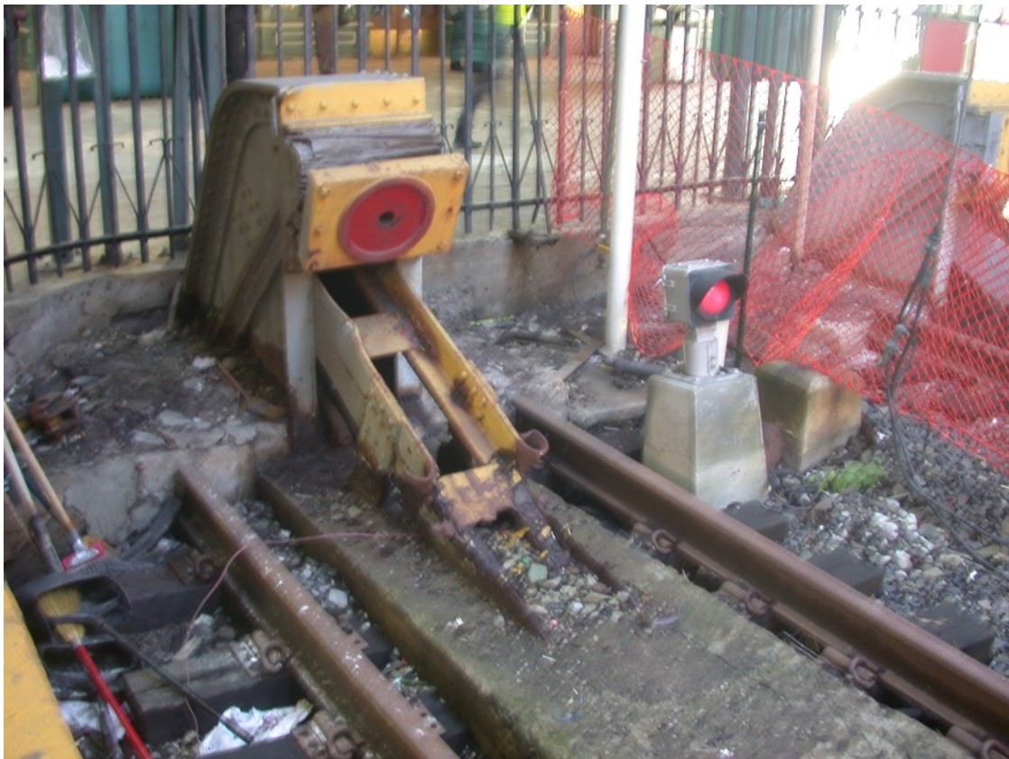
Figure 1. Photograph of an exemplar bumping post at the Hoboken Terminal.
