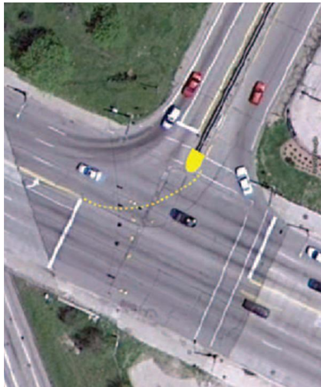
Figure 16. Example of channelization methods for a paired controlled-access highway ramp location, including a painted island and a left-turn marking extension from the crossroad. (Courtesy of the Federal Highway Administration.)
