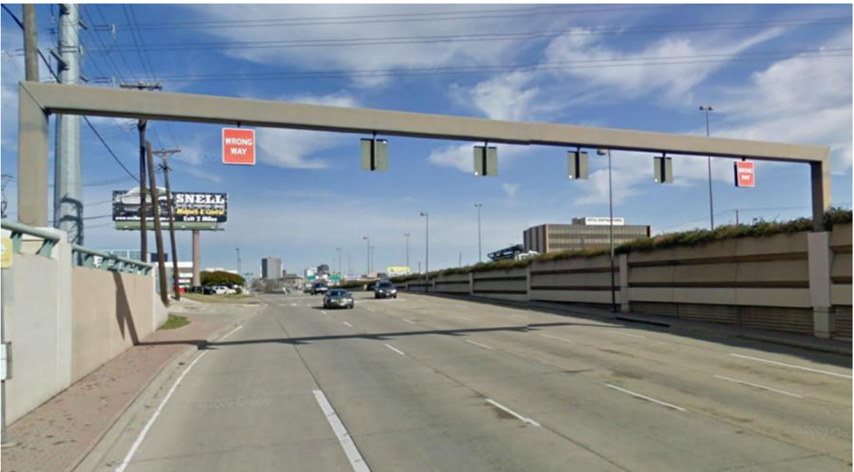
Figure 7. Mounting height of wrong-way signs on frontage road adjacent to US Highway 75 in Dallas, Texas.
