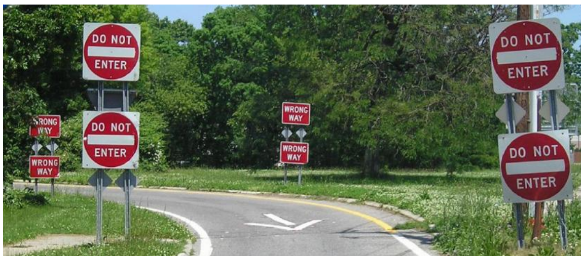
Figure 17. Double-posted “Do Not Enter” and “Wrong Way” signs on an exit ramp. (Courtesy of the New York State Department of Transportation).
