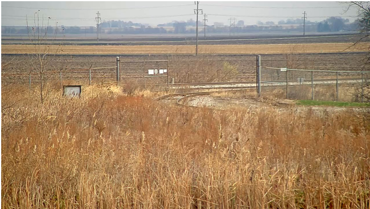
Figure 2. Gate fouling the track at the Cabot industrial facility.
