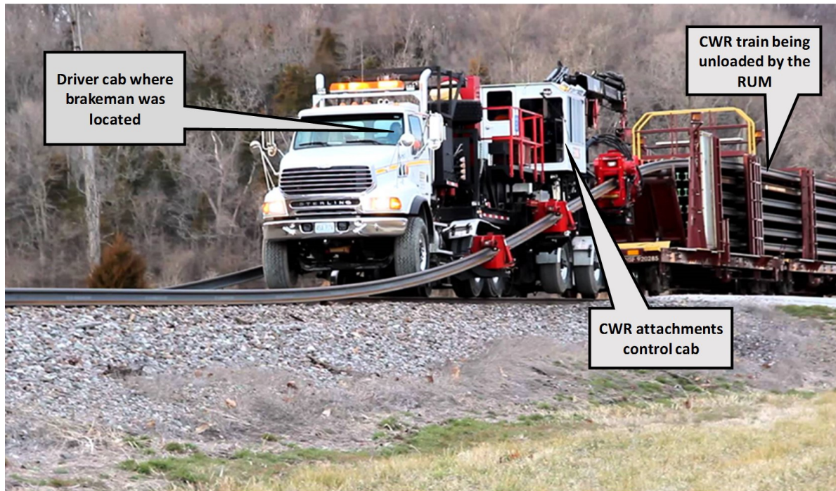
Figure 9. RUM unloading rail from CWR work train. (Source: BNSF)
