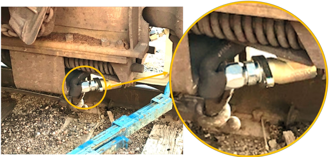
Figure 6. Kinked intermediate end-of-railcar air hose that was discovered during an inspection after an end-of-railcar air hose arrangement was incorrectly applied. (Photograph provided by UP.)
