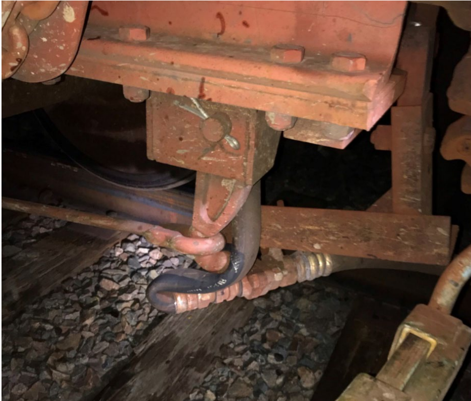
Figure 5. Kinked end-of-railcar air hose on train involved in the November 23, 2018, incident west of Cheyenne, Wyoming. (Photograph provided by UP.)
