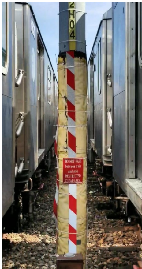
Figure 2. Postaccident identification of restricted clearance area. (Source: NYCT)
