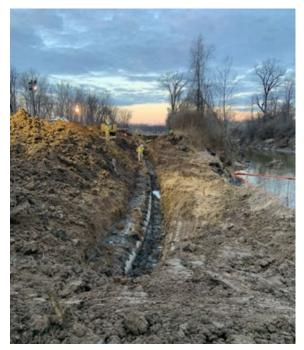
**Figure 1.** Ruptured pipeline and Cahokia Creek. (Source: Marathon.)
