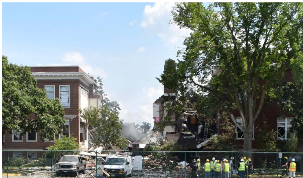
Figure 1. Photo of accident site taken after building explosion. (Source: Minneapolis Fire Department.)
