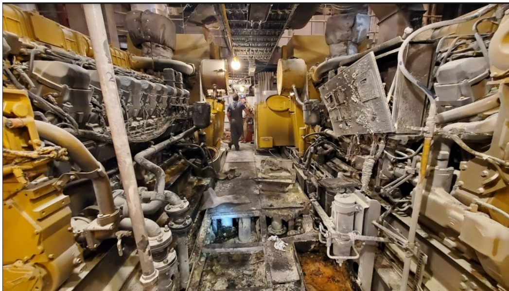
Figure 5. The walkway between the nos. 3 and 4 main engines after the engine failure (looking forward).
