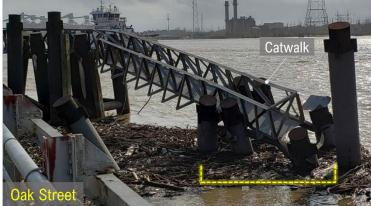
**Figure 7.** Damage to the river intake fender systems: (*left*) arrow shows damage to the spud barge at New River; (*right*) bracket identifies the damaged catwalk and dolphin piles at Oak Street downriver. (Source: Coast Guard [right photo])
