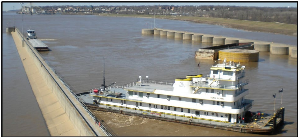
Figure 1. Kevin Michael under way at the Melvin Price Locks and Dam after the casualty. (Source: US Coast Guard)
