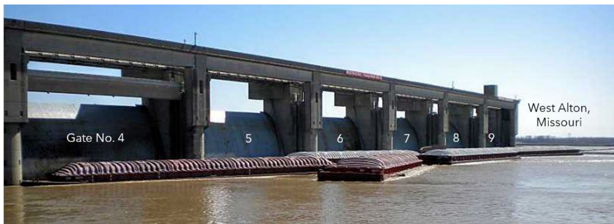
Figure 7. Barges upstream of the Melvin Price Locks and Dam west of the guide wall following the casualty. (Source: Coast Guard)
