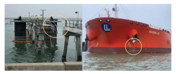
**Figure 6.** Damage to the no. 4 Moda dock catwalk (*left*) and the *Riverside* (*right*), circled. (Source: US Coast Guard)
