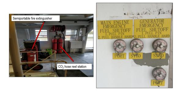
**Figure 4.** Engine room fire-extinguishing equipment (*left*). Emergency fuel oil shutoff pull station (*right*). (Source: WRBM)
