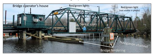
Figure 3. Centerville Turnpike Bridge in the closed position. (Source: City of Chesapeake)
