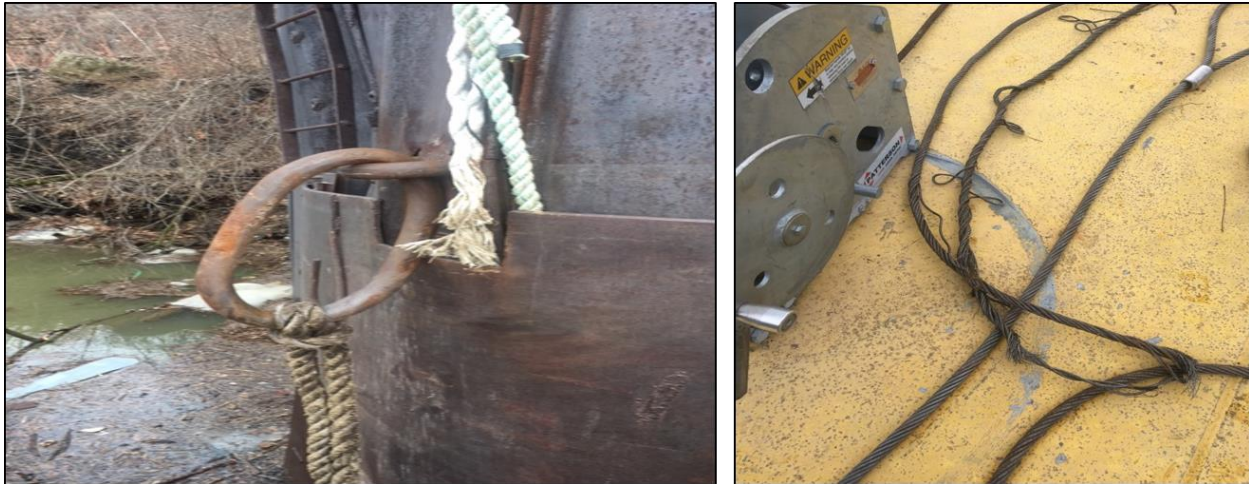
At left, a deformed anchor ring on third piling back from the forward piling. At right, parted and frayed mooring wires from the lead shore-side barge during the accident.
