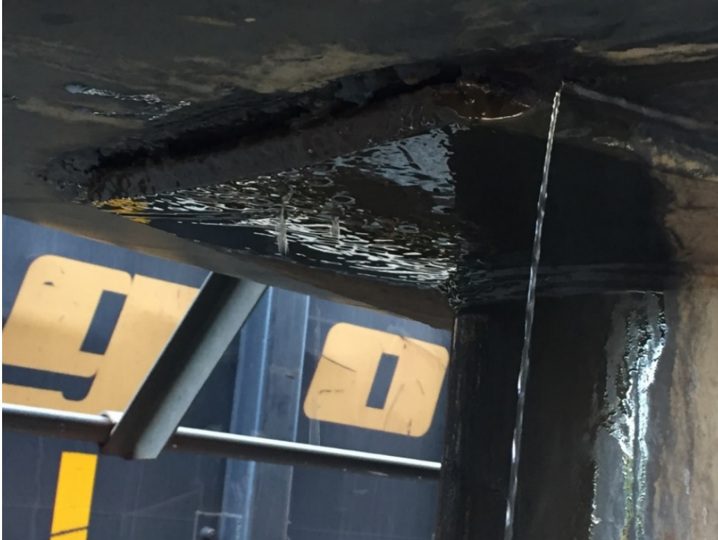
Figure 3. Ethanol leaking from the cracked tank shell. (Photograph courtesy of CSX.)
