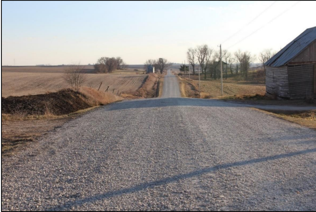
Figure 14. Gravel surface of 480th Street at crash location (looking south), with embankment on left and driveway on right.
