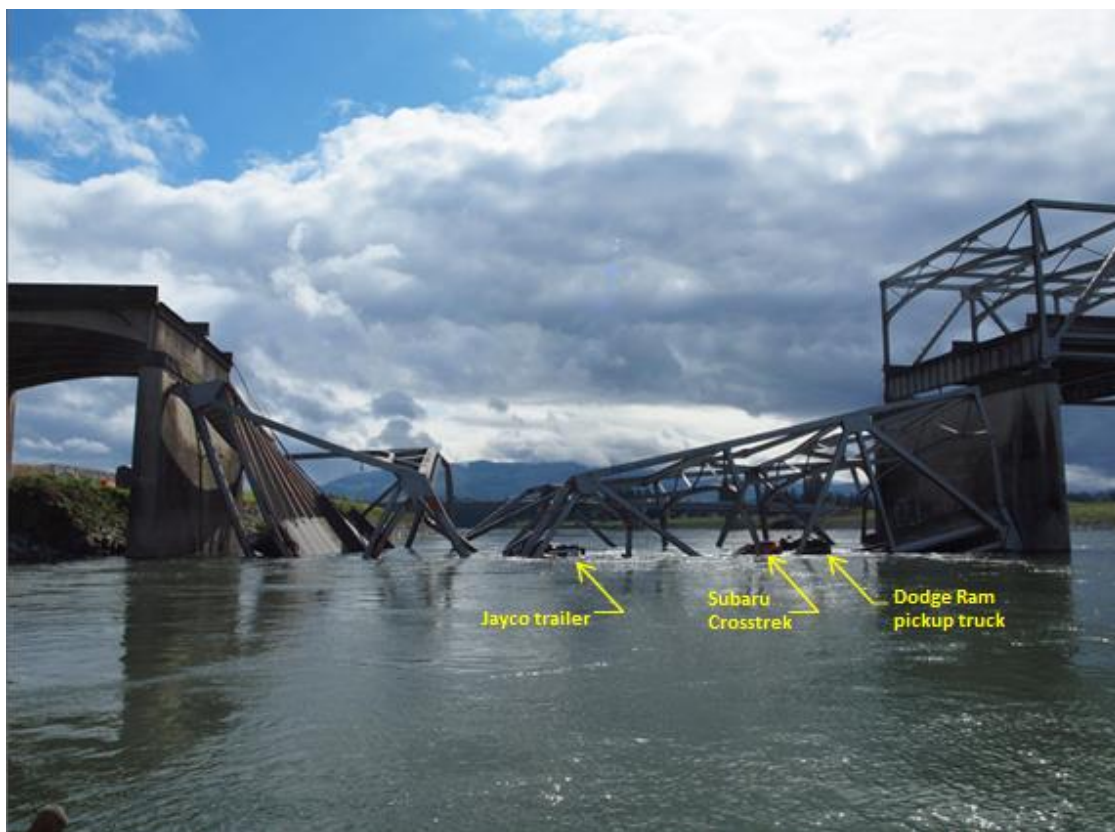
Figure 6. Bridge span 8 in the Skagit River.
