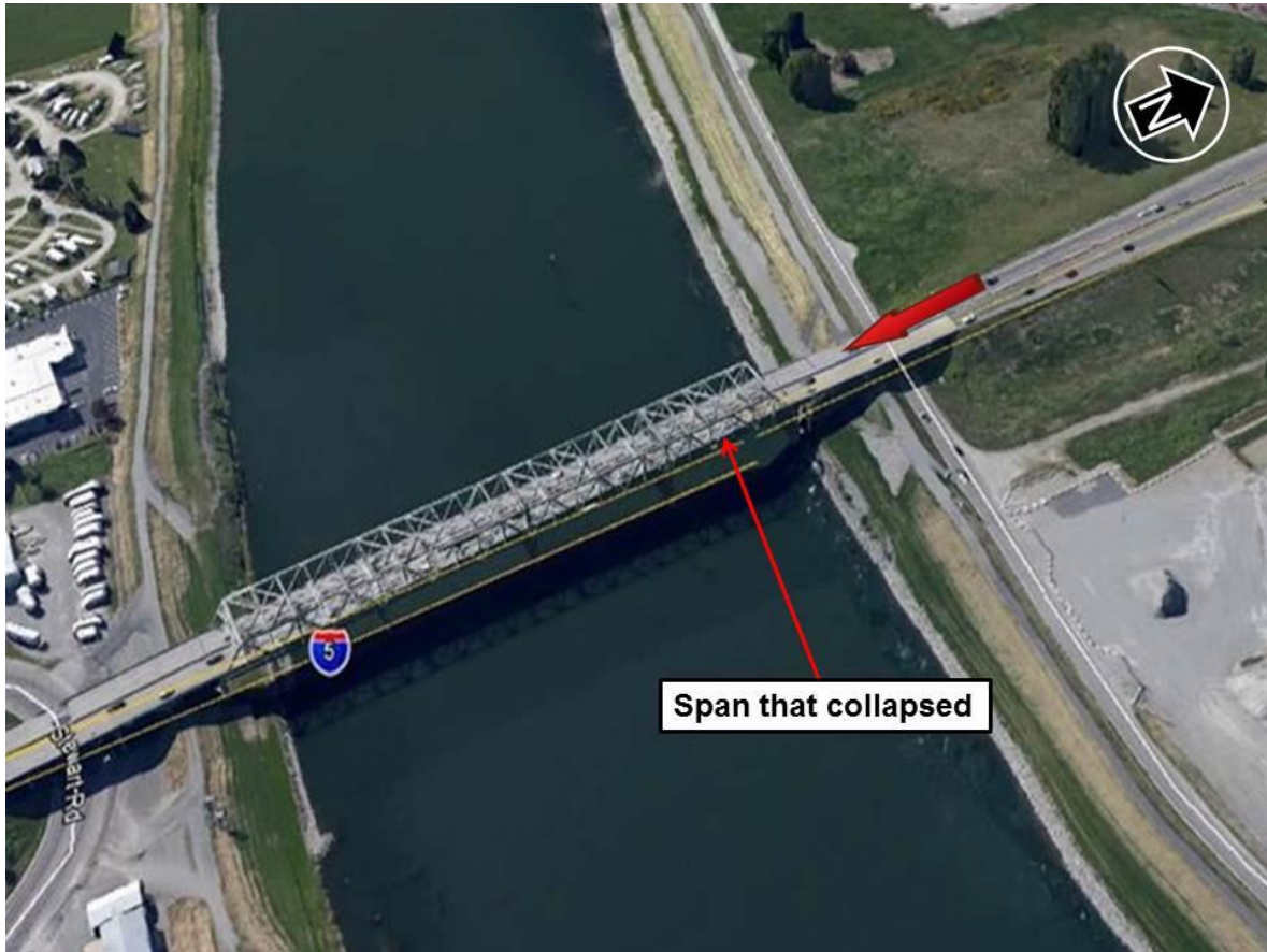
Figure 4. Aerial view, looking west, at the Skagit River (through-truss) Bridge before the span collapse. The span that collapsed is labeled, and the large red arrow shows the southbound direction of travel of the oversized combination vehicle. (Image captured by Google Earth.)
