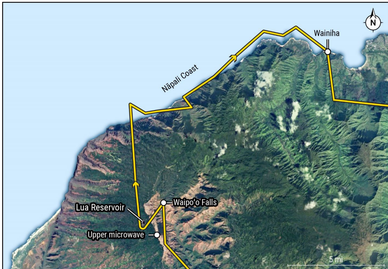
Figure 3. Upper microwave tower site.
