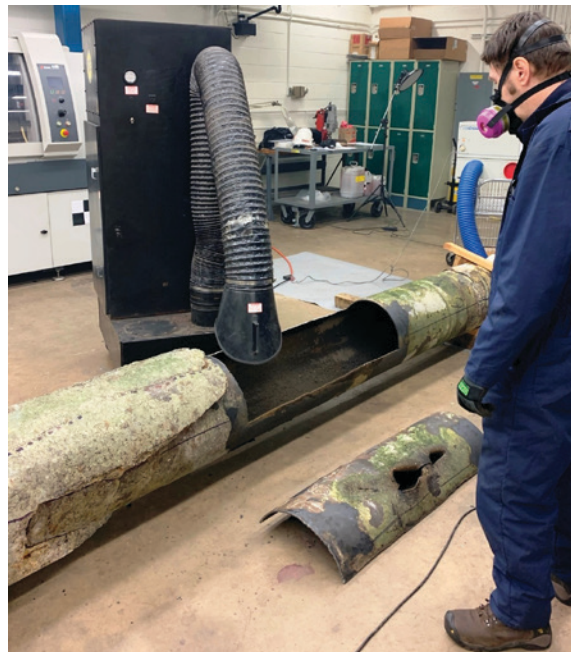
Figure 24. Materials Laboratory Division staff member removing the damaged portion of the pipe struck by dredging vessel Waymon Boyd in Corpus Christi, Texas, August 21, 2020.
