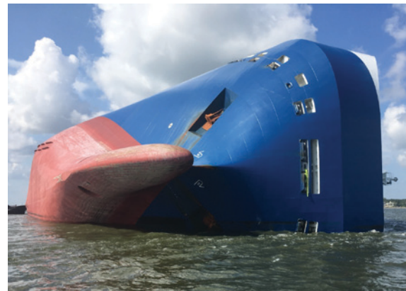
Figure 12. The Golden Ray settled at an angle of 90° after heeling quickly to port following a turn.
