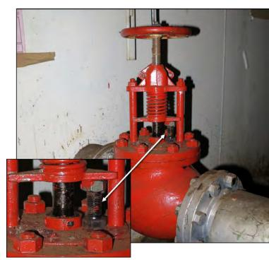
Figure 58. Postaccident photo of *Caribbean Fantasy's* quick-closing valve for the starboard heavy fuel oil storage tank that was blocked open with a bolt and nut.
