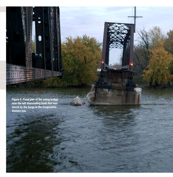
bout 0230 on October 26, 2017, the towing vessel *Cooperative Venture*, with a crew of 10, was pushing 12 barges downbound on the Mississippi River near St. Paul, Minnesota. As the vessel approached the St. Paul Union Pacific Rail Bridge at mile 835.7, the lead barge on the port side struck a fixed pier of the swing bridge. There were no reported injuries or pollution. Damages to the bridge and barge were estimated at \$800,000 and \$153,000, respectively.
