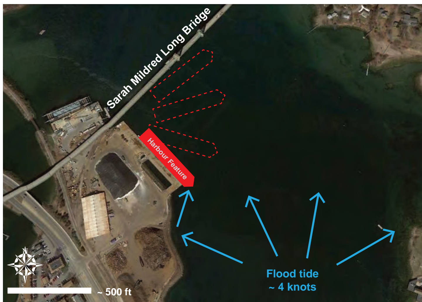
Aerial view of the Marine Terminal Wharf on the Piscataqua River. The overlaid blue arrows illustrate the direction of the strong flood current. The overlaid orange-red icons illustrate how the Harbour Feature moved toward the bridge after the mooring lines parted. (Background by Google Earth)
