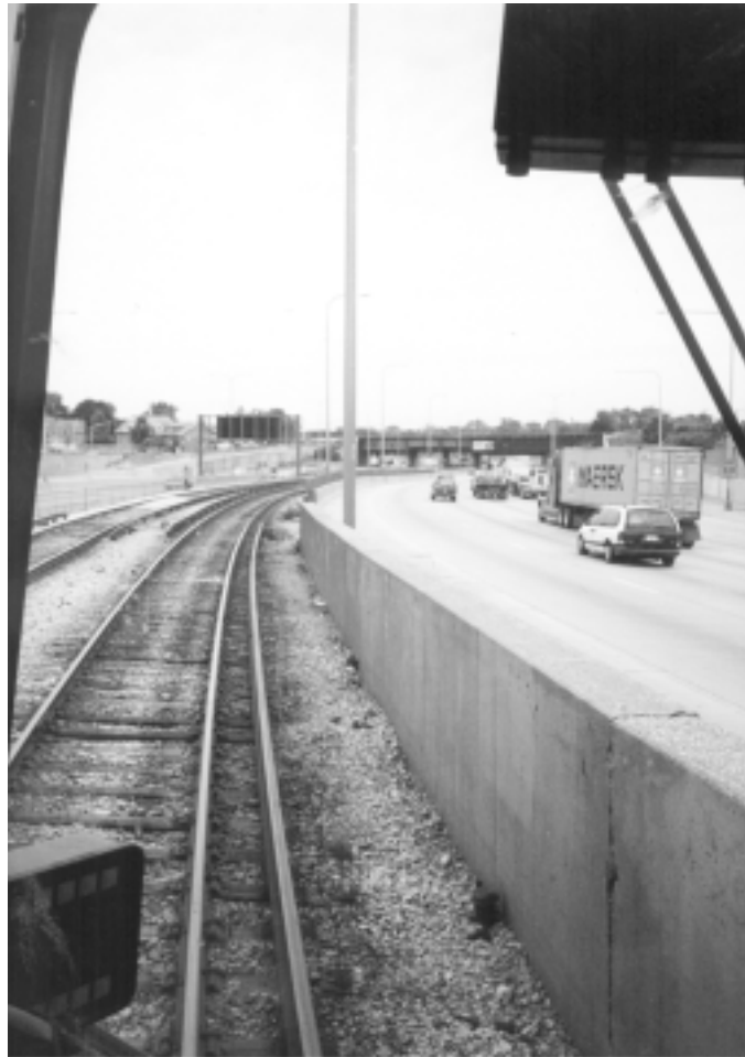
Figure 3. Operator's view as train approaches June 17 accident location.
