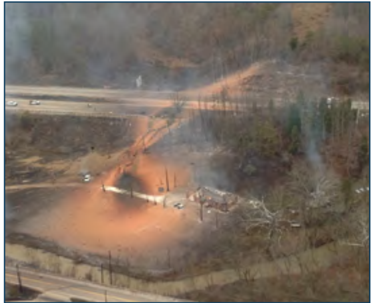
Aerial photo of the damage from the December 11, 2012, pipeline rupture that occurred west of I-77 near Sissonville, West Virginia.
