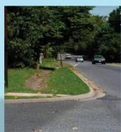
A sidewalk ends at a driveway without providing an accessible connection to the walkable shoulder in the distance. Pedestrians, especially during and after rain storms, are forced to walk in the right turn lane as the landscaped area between facilities is sloped toward the open channel. The RSA team may provide suggestions for improving the safety of this connection.
