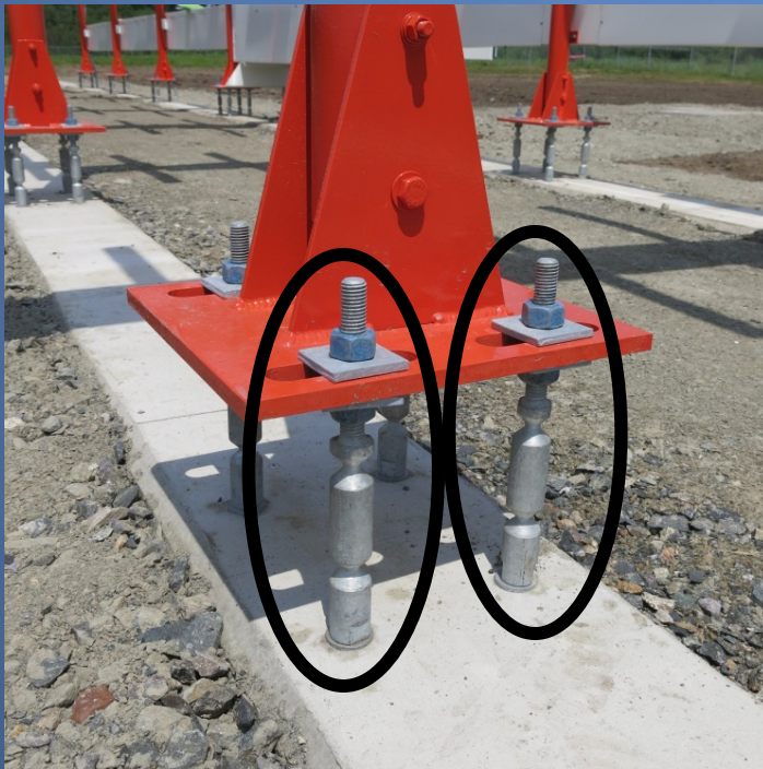
Frangible localizer antenna support
