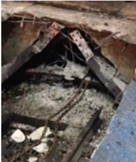
Figure 5. Destroyed bumping post.
