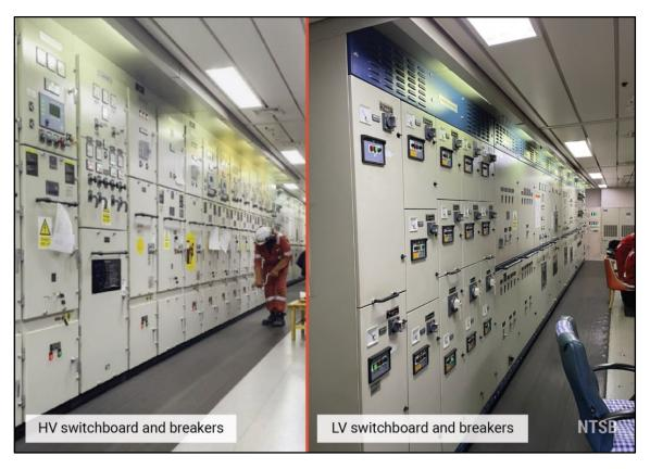
**Figure 3.** The *Dali*'s power management system in the ship's engine control room. The HV switchboard (which houses the HV bus) and breakers (*left*) and the LV switchboard (which houses the LV bus) and breakers (*right*).
