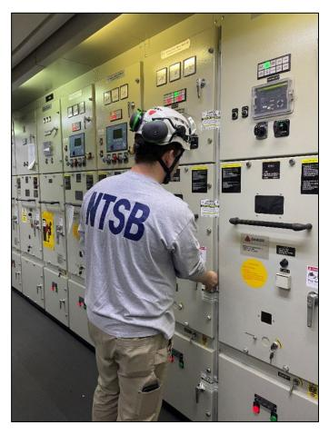
**Figure 8.** An NTSB investigator examining the *Dali's HV* switchboard (which houses the HV bus) and applying tamper-evident preservation seals.
