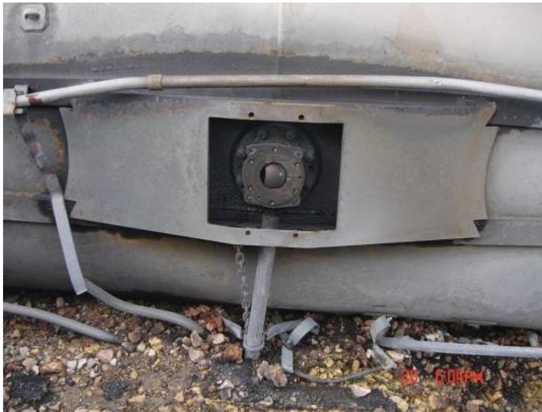
Figure 12. Bent valve handle and exposed and partially open bottom outlet valve on car NATX 303504. (Federal Railroad Administration photo)
