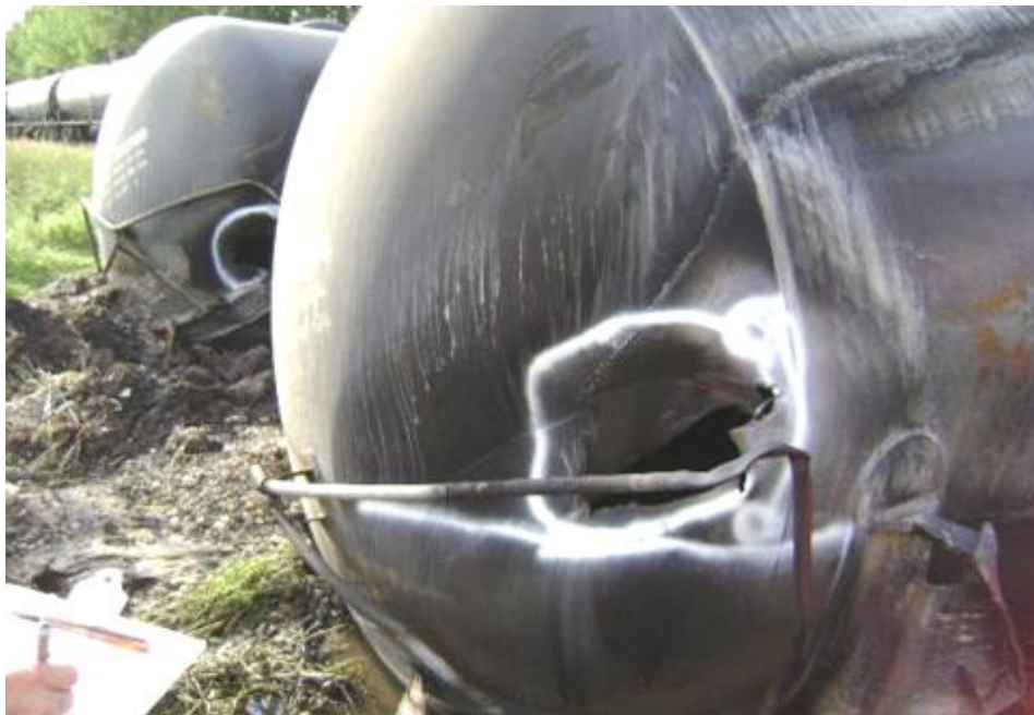
Figure 9. Tank head punctures in two derailed tank cars (outlined with white paint). (Federal Railroad Administration photo)
