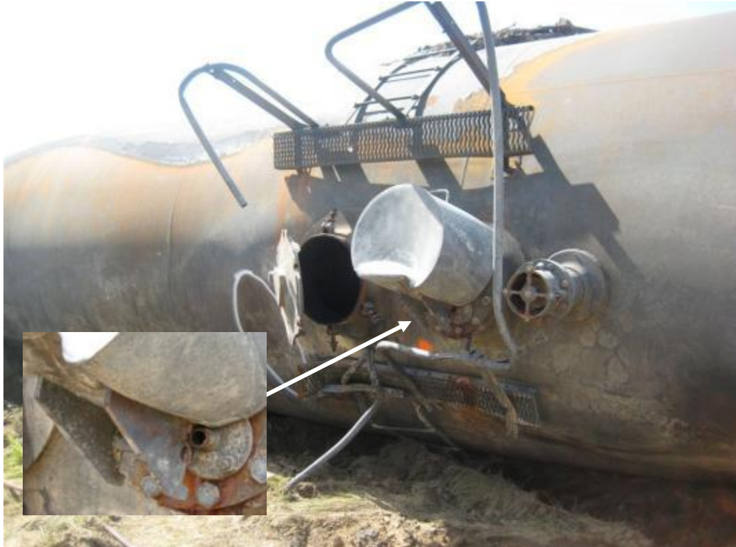
Figure 13. Top fitting damage, car TILX 193772. (Overall photo by Trinity Tank Car. Inset photo by the CN.)
