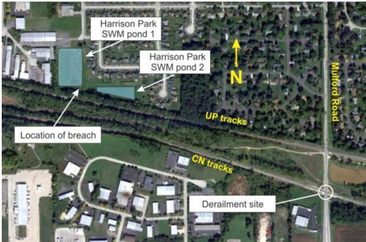
Figure 15. Aerial view showing location of Harrison Park subdivision detention ponds in relation to accident site.
