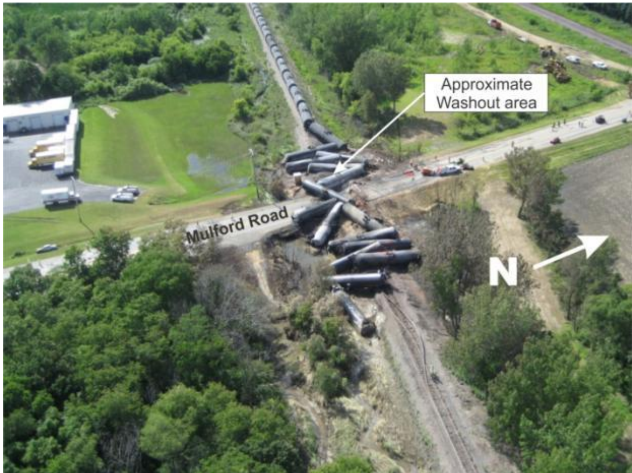
Figure 3. Aerial view, looking northwest, of derailed tank cars after locomotives and first 58 cars have been pulled away from wreckage.
