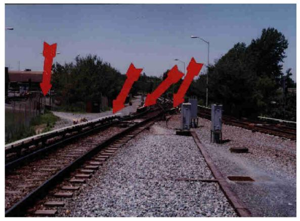
Figure 11 -- Looking north toward the interlocking just north of the Shady Grove passenger station. Arrows at center indicate portions of third rail that remained energized for approximately 40 minutes after the accident. Arrow at left indicates property security gate through which rescue workers entered the track bed.
