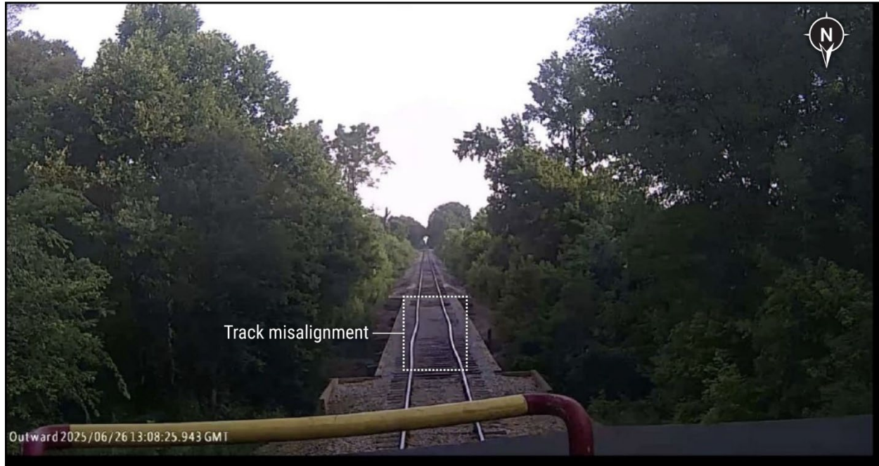
Figure 2. June 26, 2025, outward-facing camera view of derailment location. (Courtesy of GRYR.)
