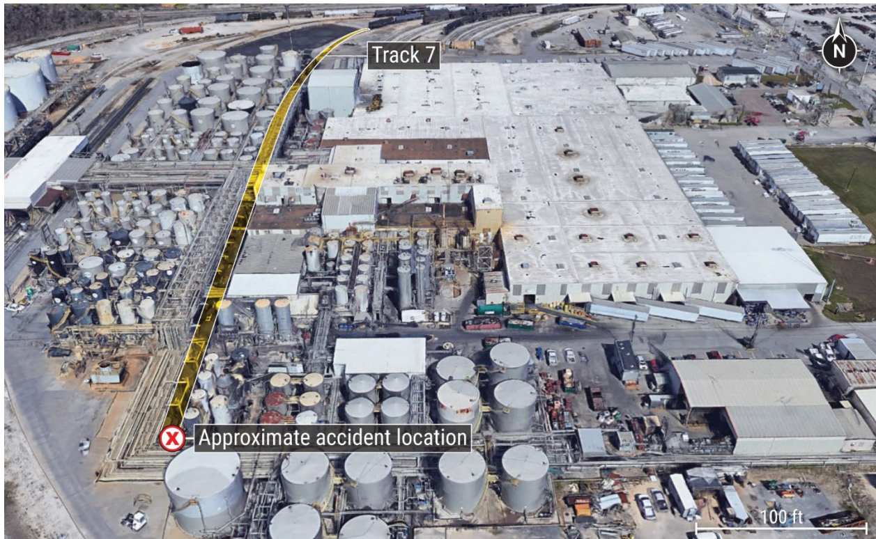
Figure 1. Overhead view of accident area.
