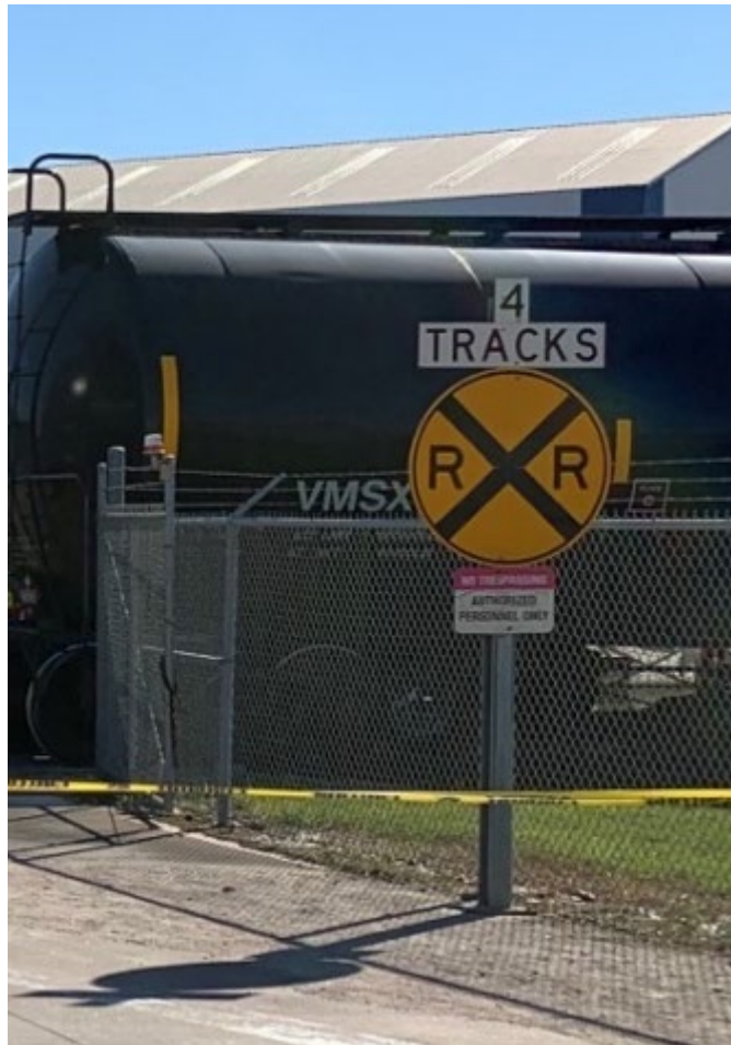
Figure 3. Highway-railroad grade crossing at Greens Port Industrial Park (Source: Federal Railroad Administration.)
