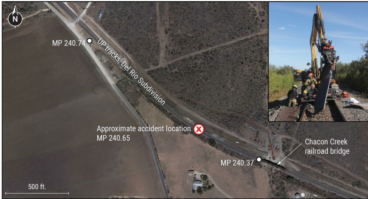
Figure 1. Overhead of accident location with a postaccident inset of the RMM. (Source: Google Earth.)
