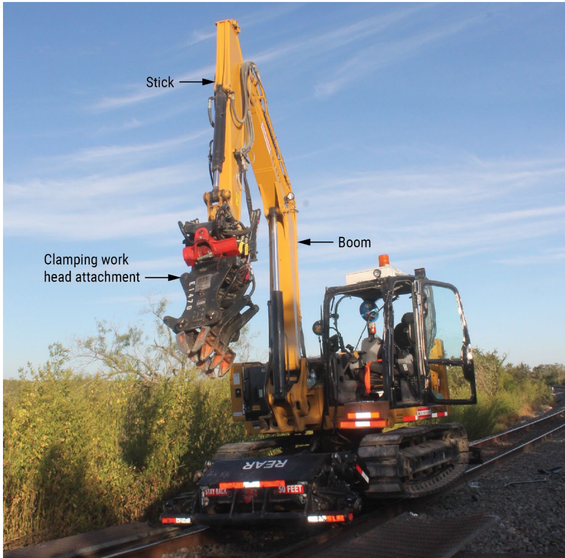
Figure 2. Accident RMM with clamping work head attachment. (Source: UP.)
