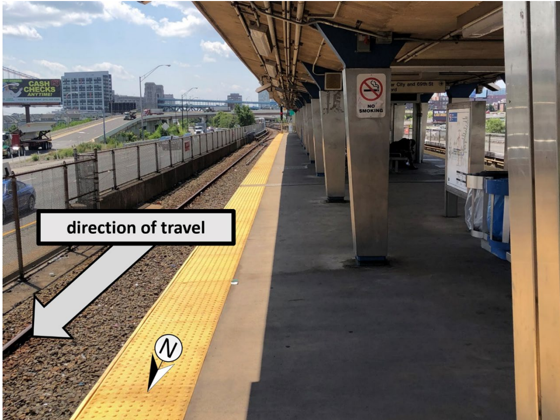
Figure 2. Spring Garden Station. (Photo courtesy of Pennsylvania Department of Transportation.)
