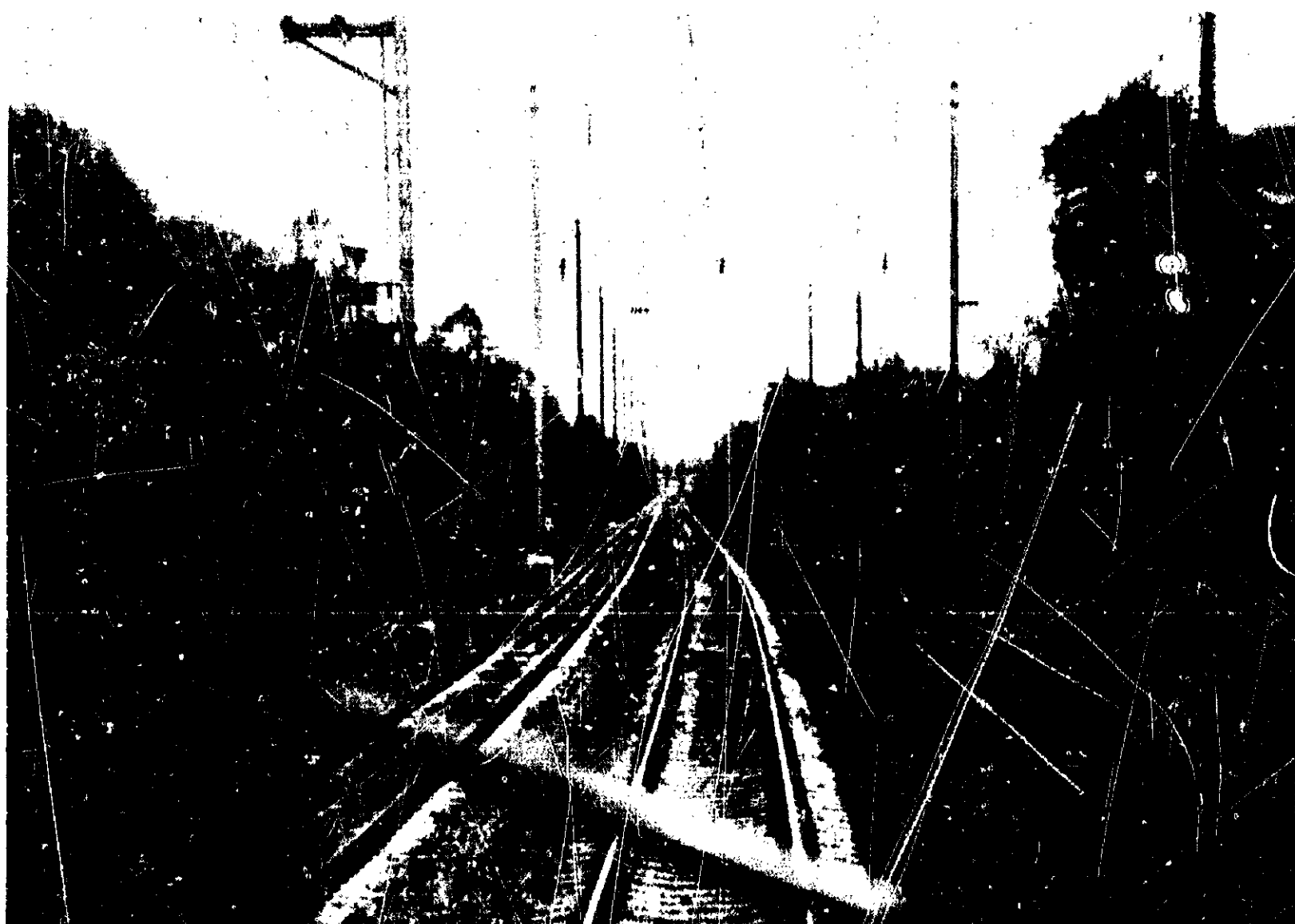
Figure 10. Code chande point CS-806 as seen from a northbound train on track 2. Th nearest catenary support poles mark the location of the code change point. The Gunpow home signals are in the distance.
