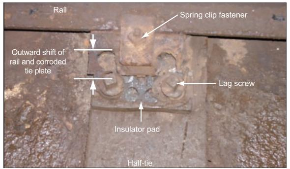
Figure 2. Outside rail of curve near point of derailment.
