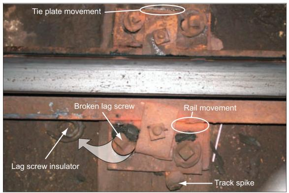
**Figure 4.** Tie plate and rail movement of outside rail near point of derailment. Large white arrow shows displacement of insulator from broken lag screw.
