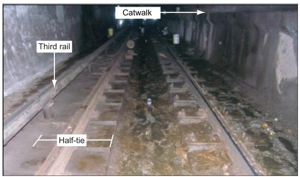
Figure 3. Chicago Transit Authority subway tunnel in derailment area, showing mud and water conditions.
