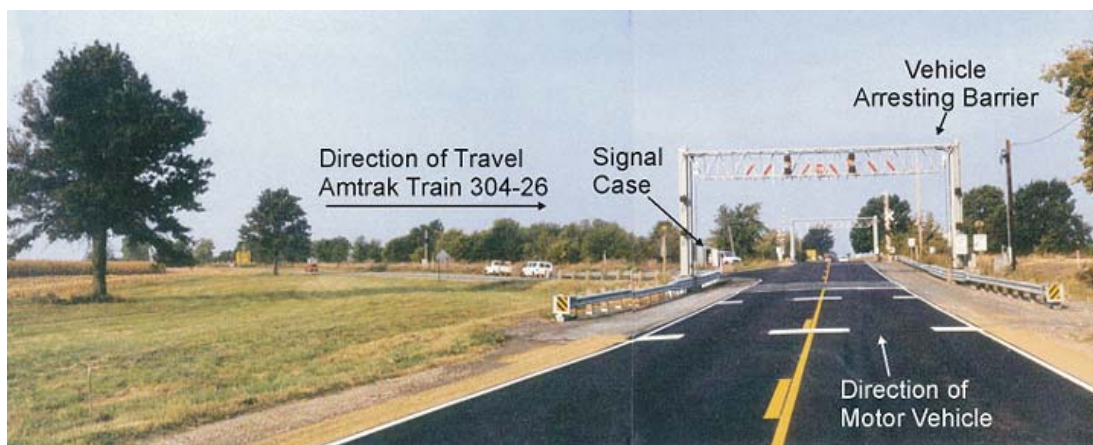
Figure 5. View down tracks from accident vehicle's direction of travel.
