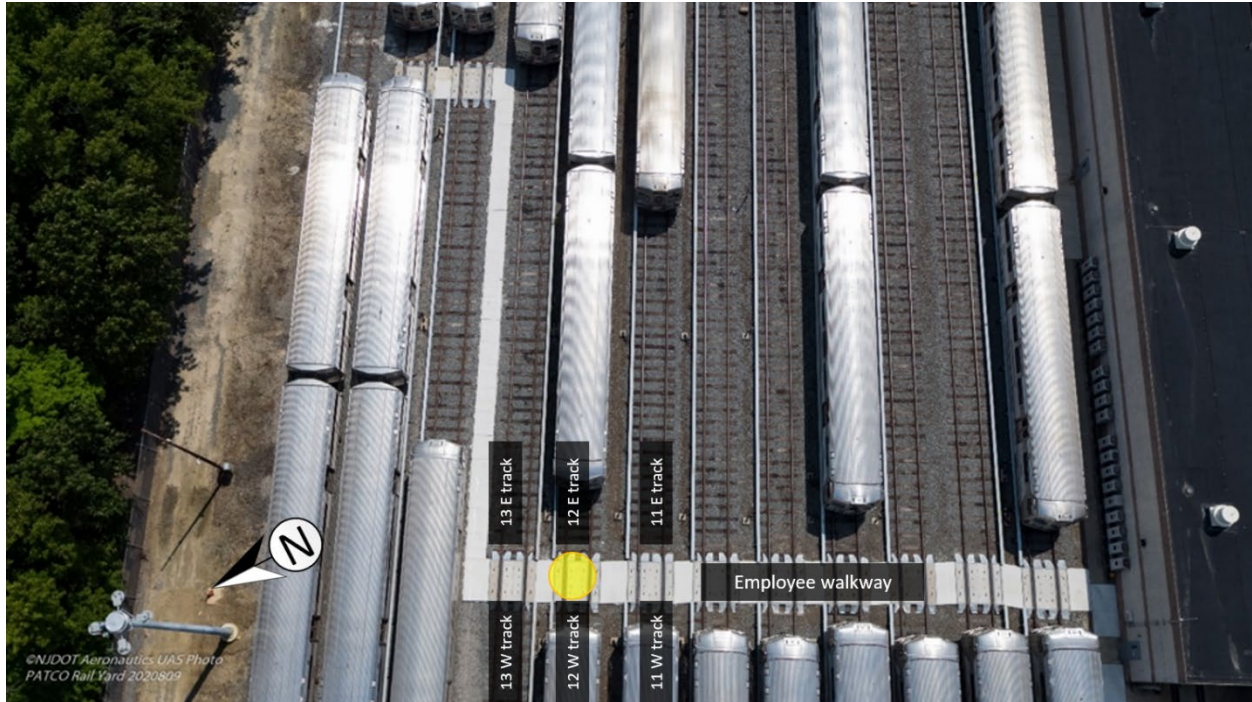
Figure 1. Aerial photograph of employee walkway. (Photo courtesy of New Jersey Department of Transportation.)
