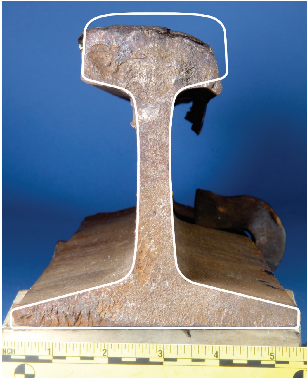
Figure 4. Excessive rail head wear on a 90-pound rail from the Aberdeen Subdivision.
