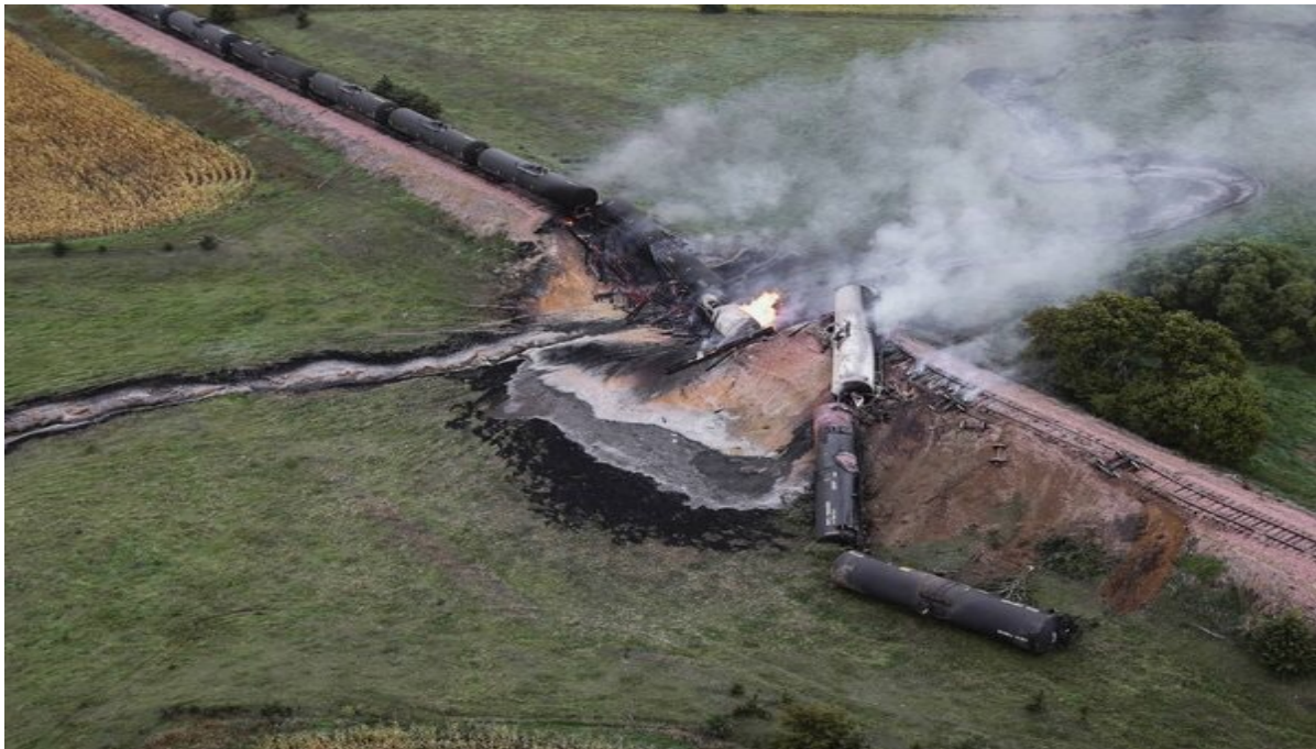
Figure 1. The accident site. (Photograph provided by BNSF.)
