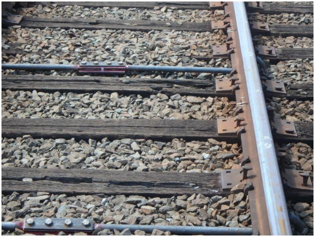
Figure 2. Deteriorated crossties at accident location. The gage rods were added postaccident.
