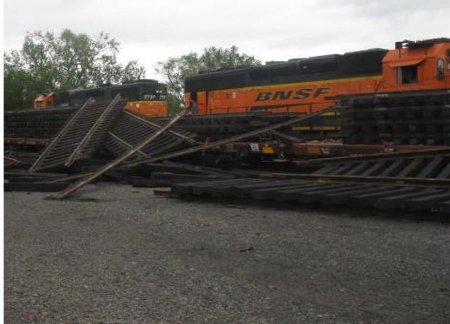
Figure 3. Dislodged track panels. (Photo: BNSF Railway)
