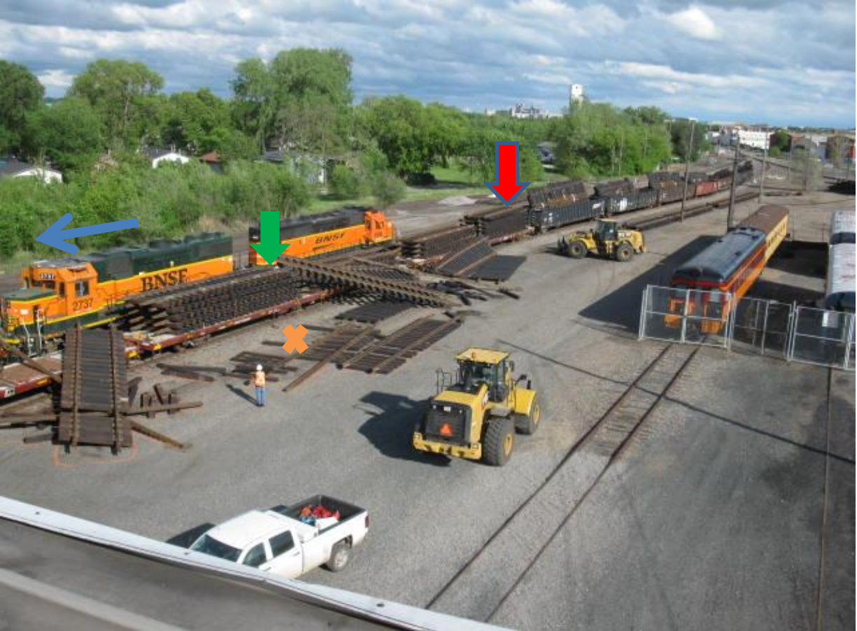
Figure 1. In this postaccident photo, the red arrow shows the fork lift operator’s position when he tried to lift two track panels. The green arrow shows the foreman’s likely position. The blue arrow indicates the direction of the train; “X” shows the location of the deceased. (Photo: BNSF Railway)
