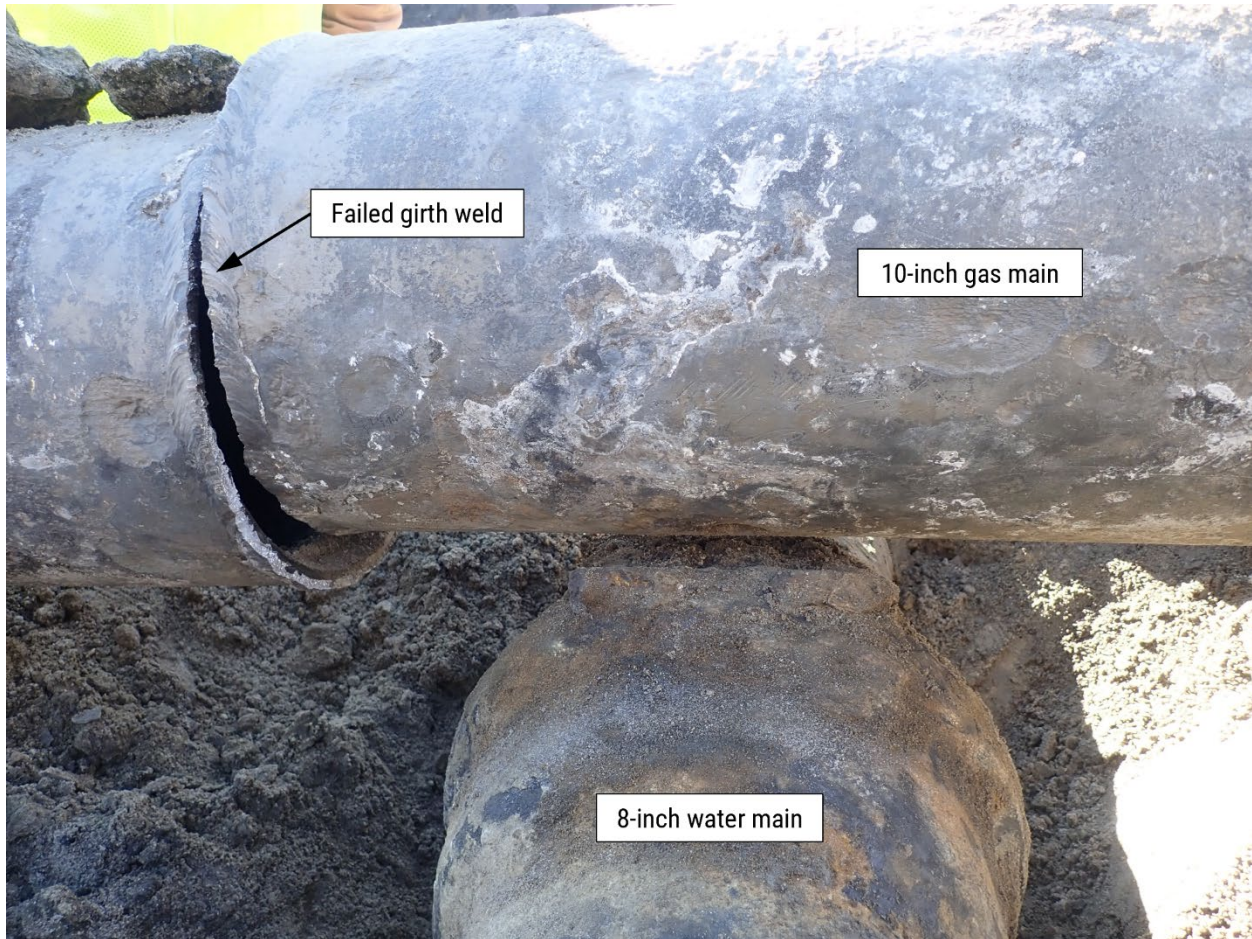
Figure 2. Ten-inch diameter gas main girth weld crossing over the 8-inch vintage water main. (Source: Baker Risk.)
