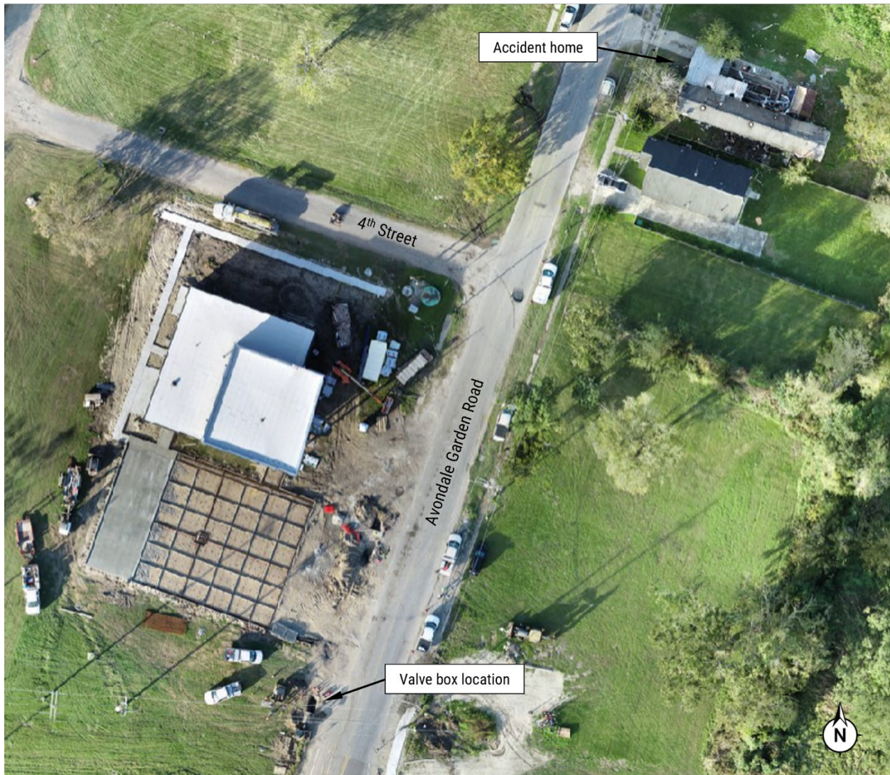
Figure 2. Overhead view of accident site. (Source: Atmos.)
