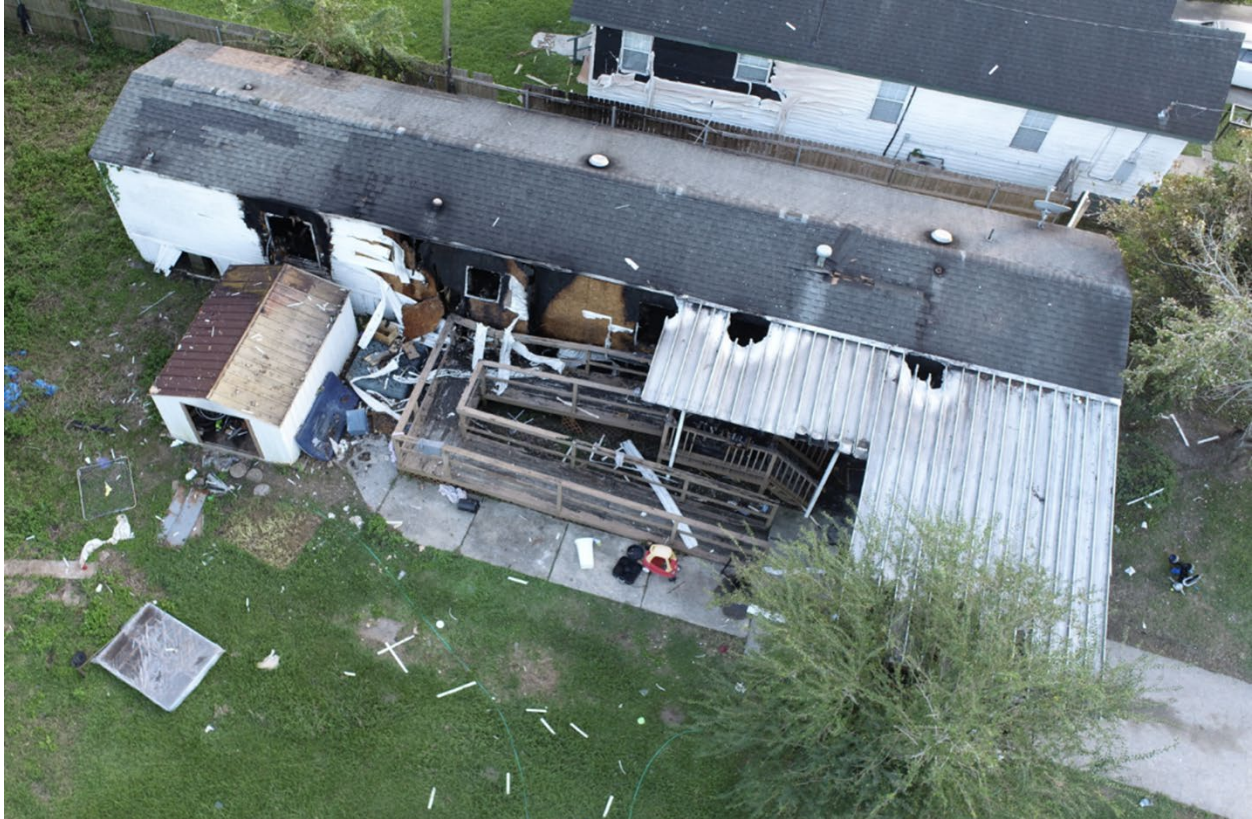
Figure 1. Accident home after the explosion and fire. (Source: Atmos.)
