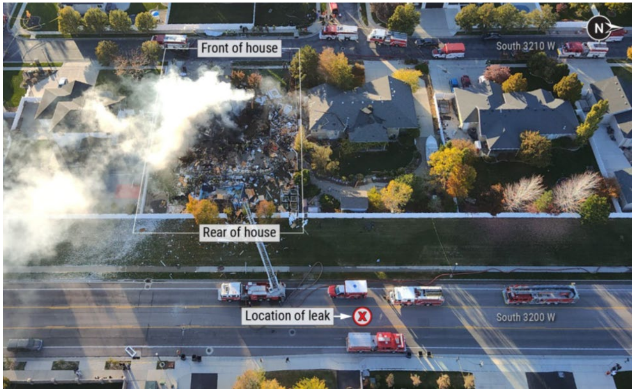
Figure 1. The scene on the day of the accident. (Drone photography courtesy of the South Jordan Police Department.)
