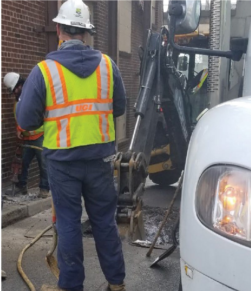
Figure 18. UGI crew during service line replacement project, 2021. (Photo courtesy Palmer.)
