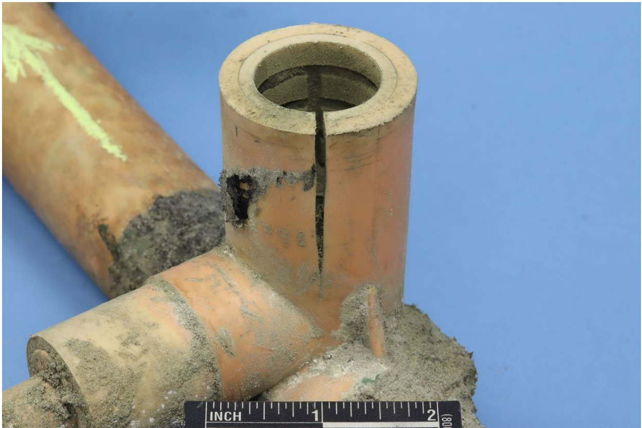
Figure 13. Longitudinal fracture in retired service tee.
